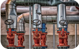
PIPELINE SYSTEM AUTOMATIC PUMPING
